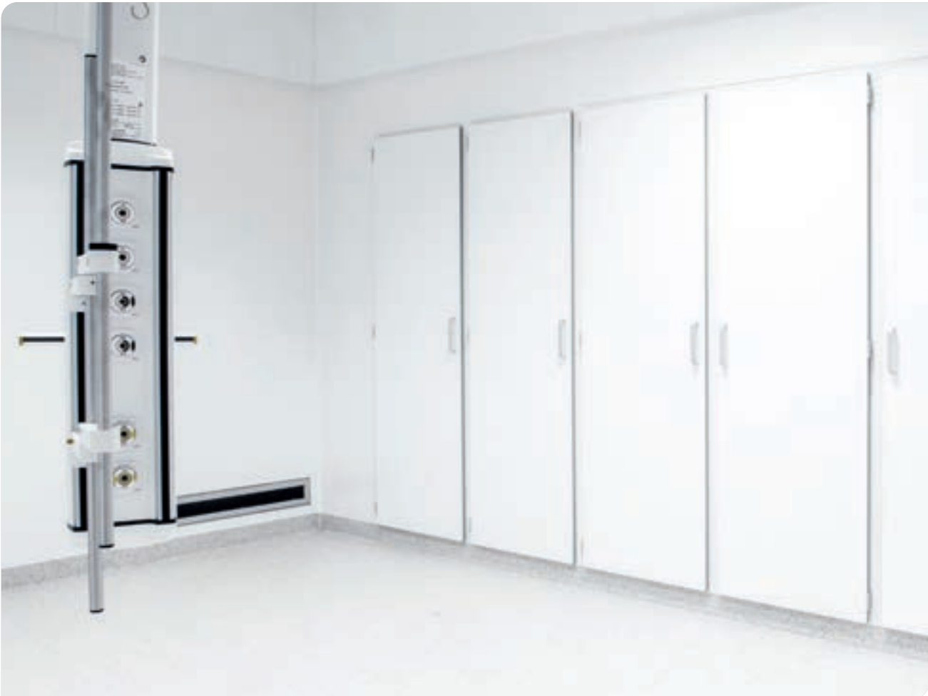
40/60 modular pass-through cabinets seen from the side of the OR room
